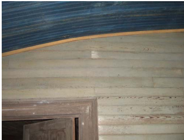
Center-passage ceiling of the Lancaster-Roach House (BW0370).
