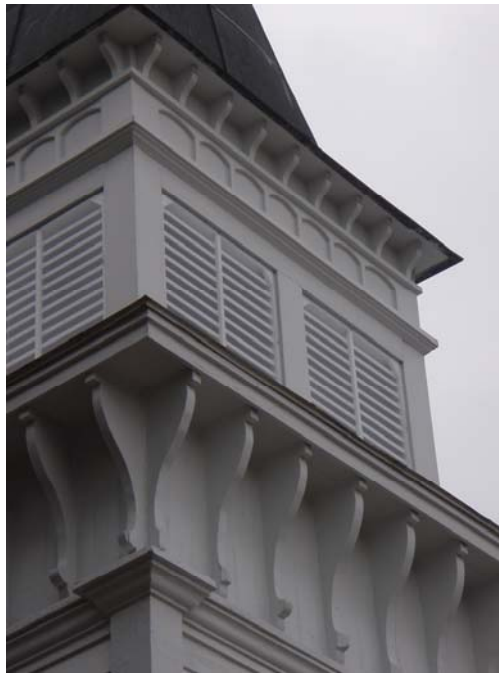
Tower of St. Philip's Episcopal Church (BW0157), Southport.
