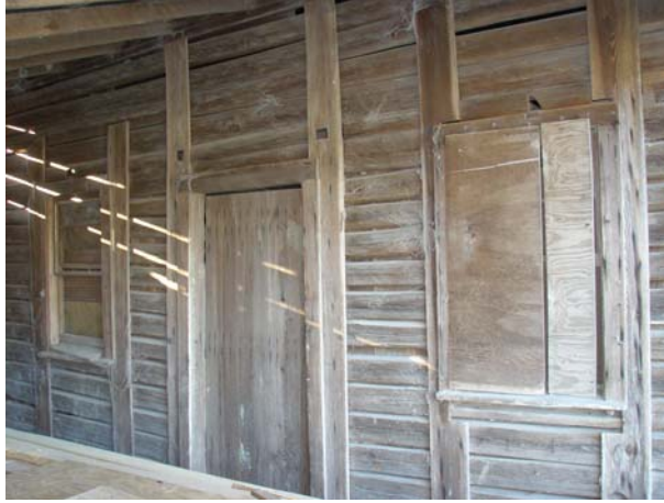
Front walls of the log house on the Ross-Smith Farm (BW0439).
