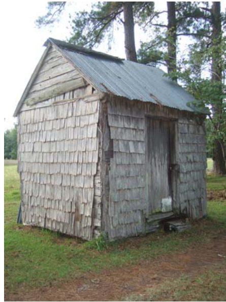
Probable dairy on the farm at 6130 Best Farm Road (BW369).
